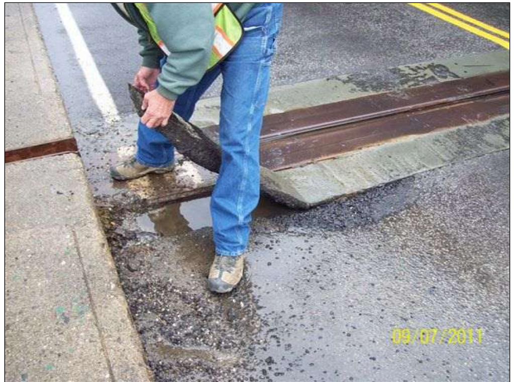
Header Peeling Up
