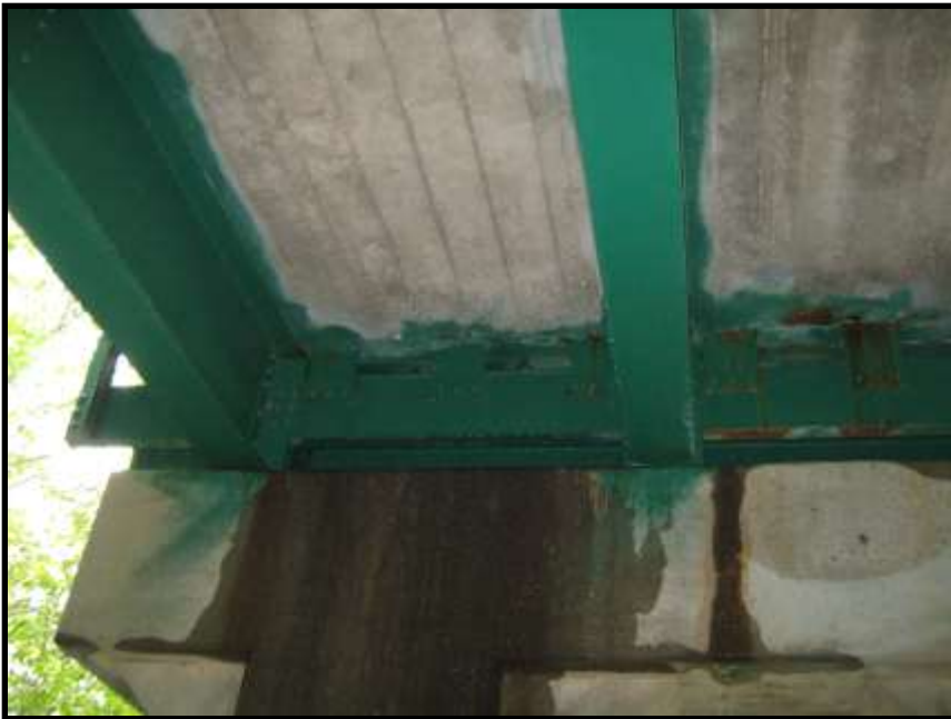
View underneath Max Wilder Bridge showing result of leaky joint seal.
