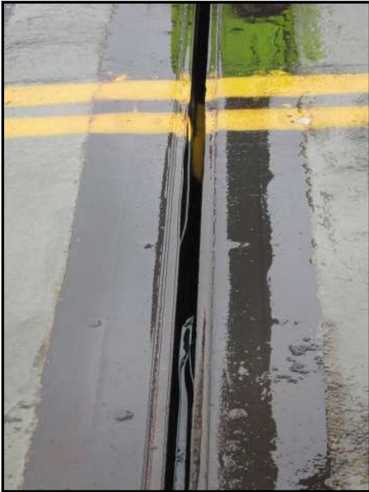
Seal Falling Out
