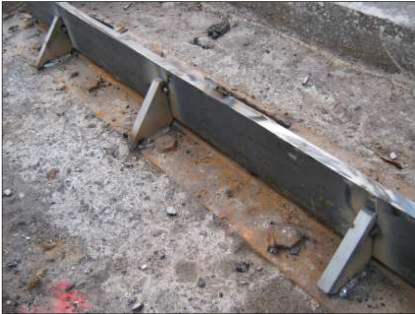
Field Modifications of Steel
