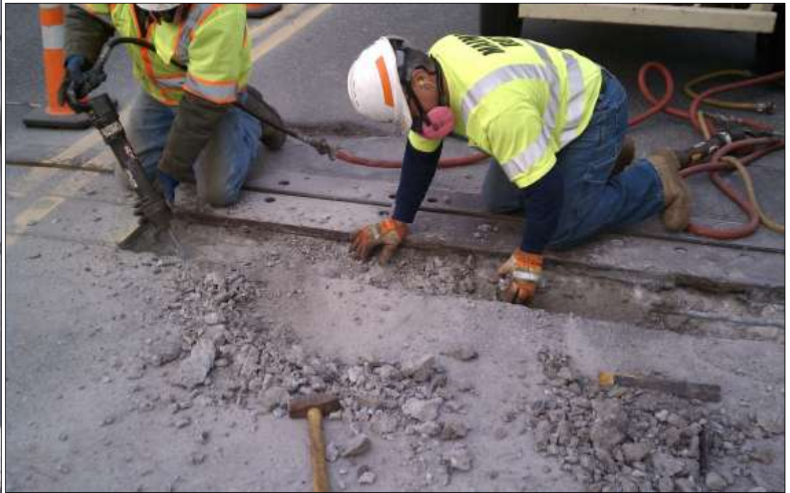
Emergency Header Repair on Frank J. Wood Bridge
