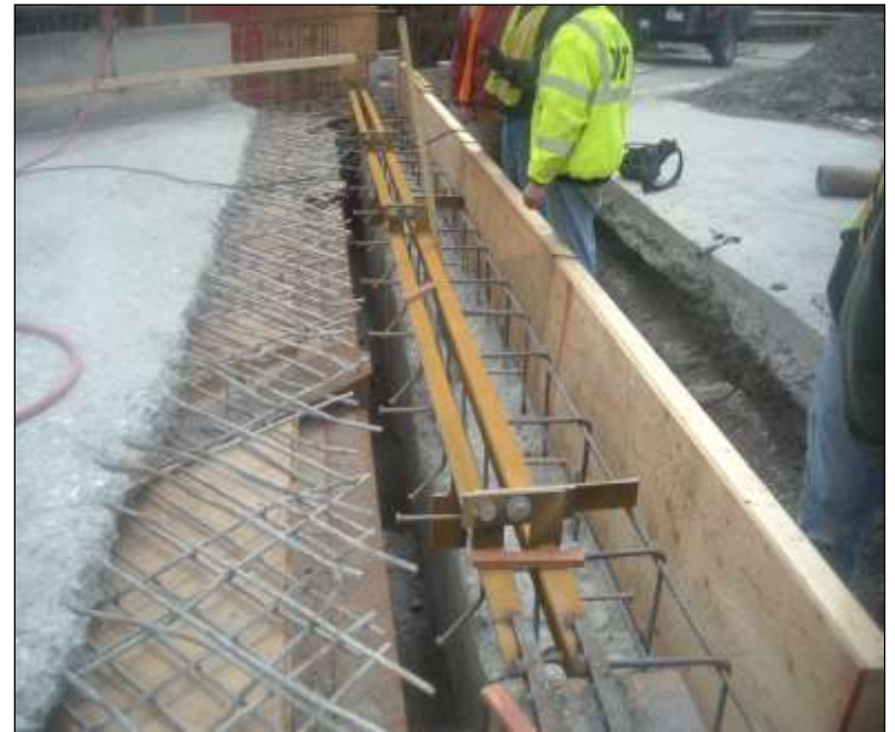
New Armored Expansion Device
