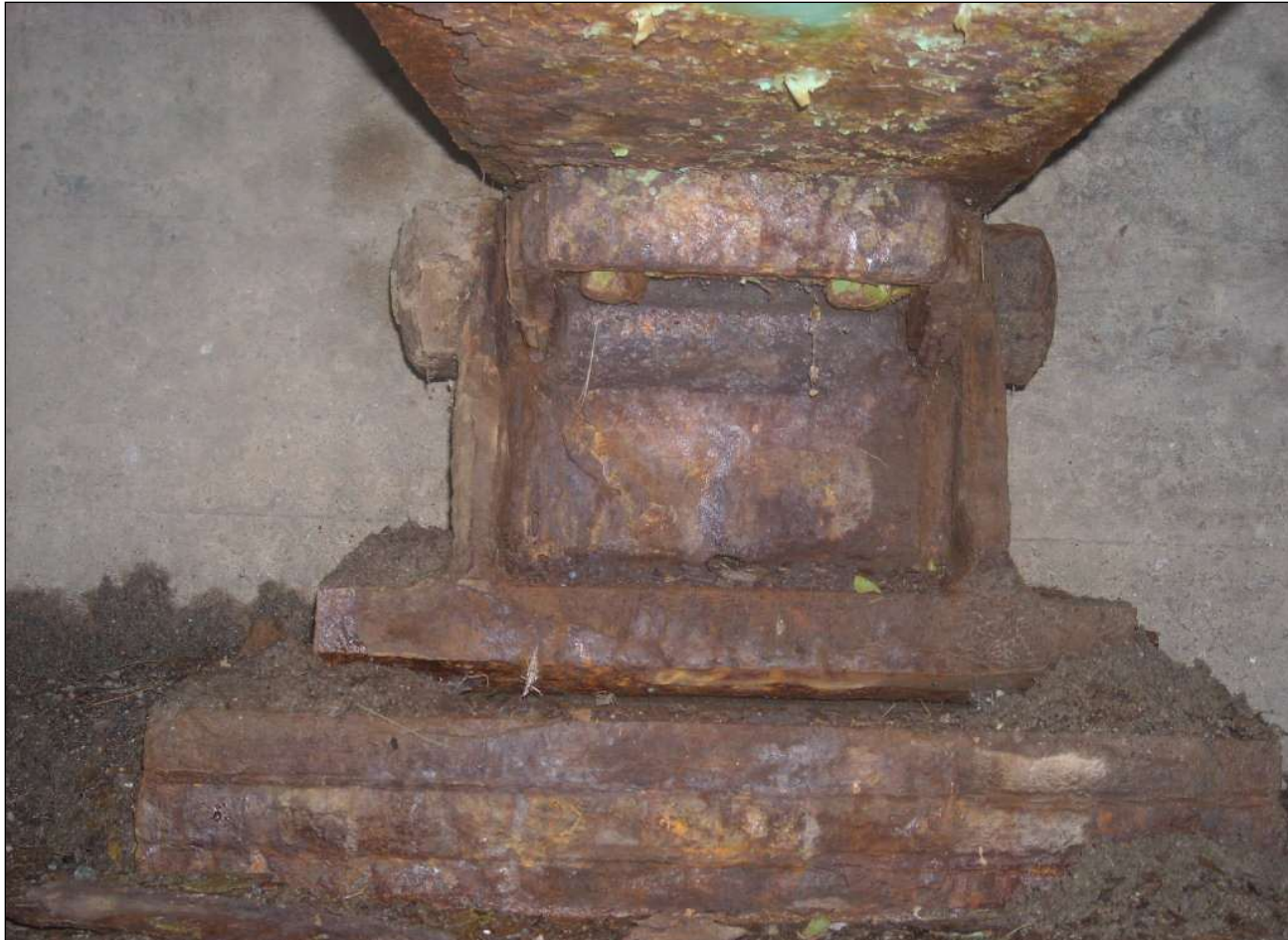
Sandy River Bridge, New Sharon
